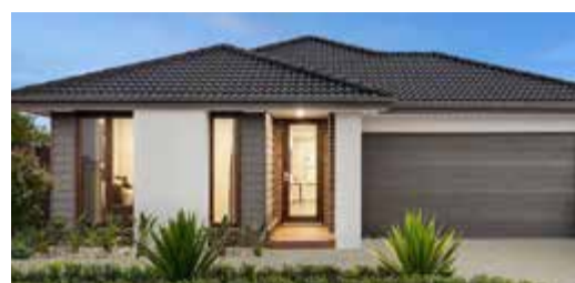
Lirello, S4 Facade — by Eight Homes
