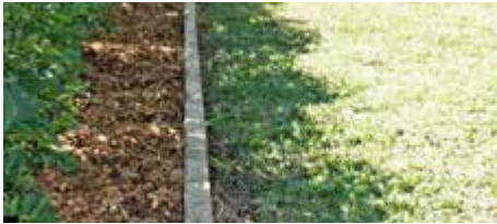
Timber edging. Treated pine garden edging or aluminium garden edging 'formboss' or similar.
