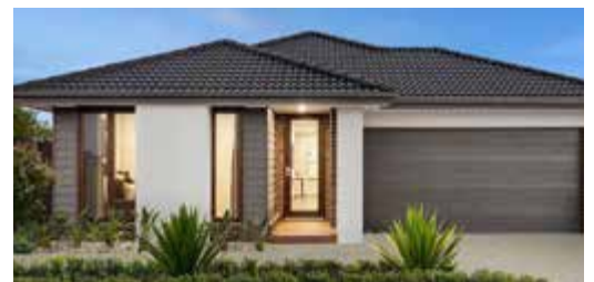
Lirello, S4 Facade — by Eight Homes
